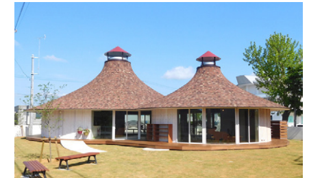
Donated windows and toilets to the "Playground-for-All" in Minamisoma as part of a recovery support project
